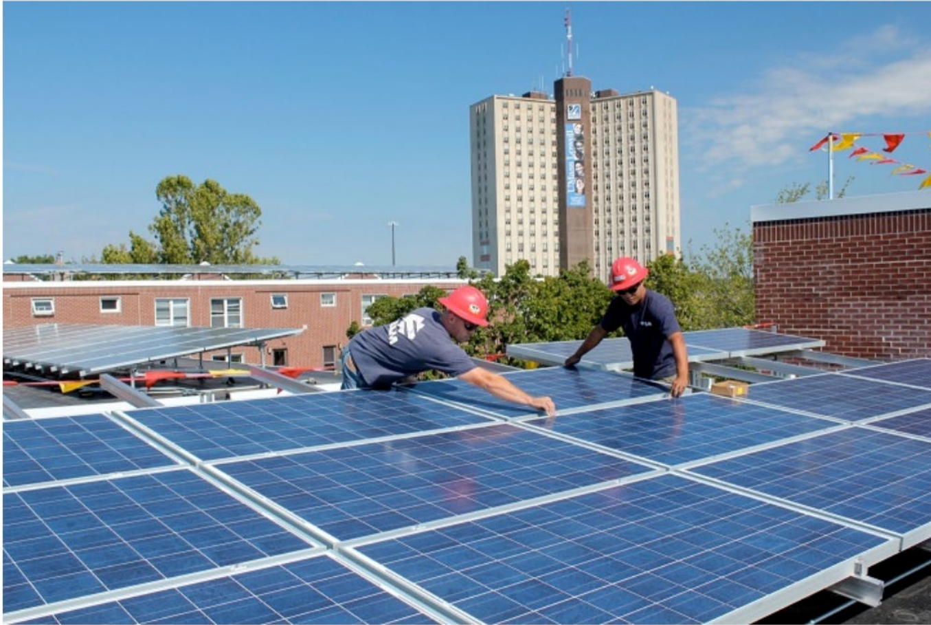
North Canal Apartments, Lowell, MA
