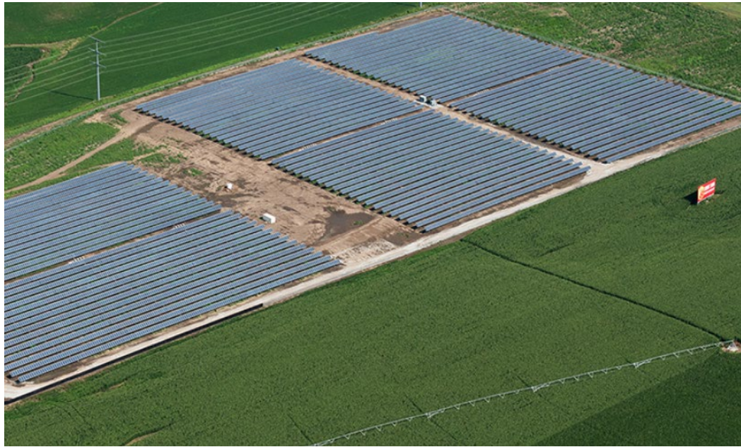
Lincoln, Nebraska + Habitat for Humanity
